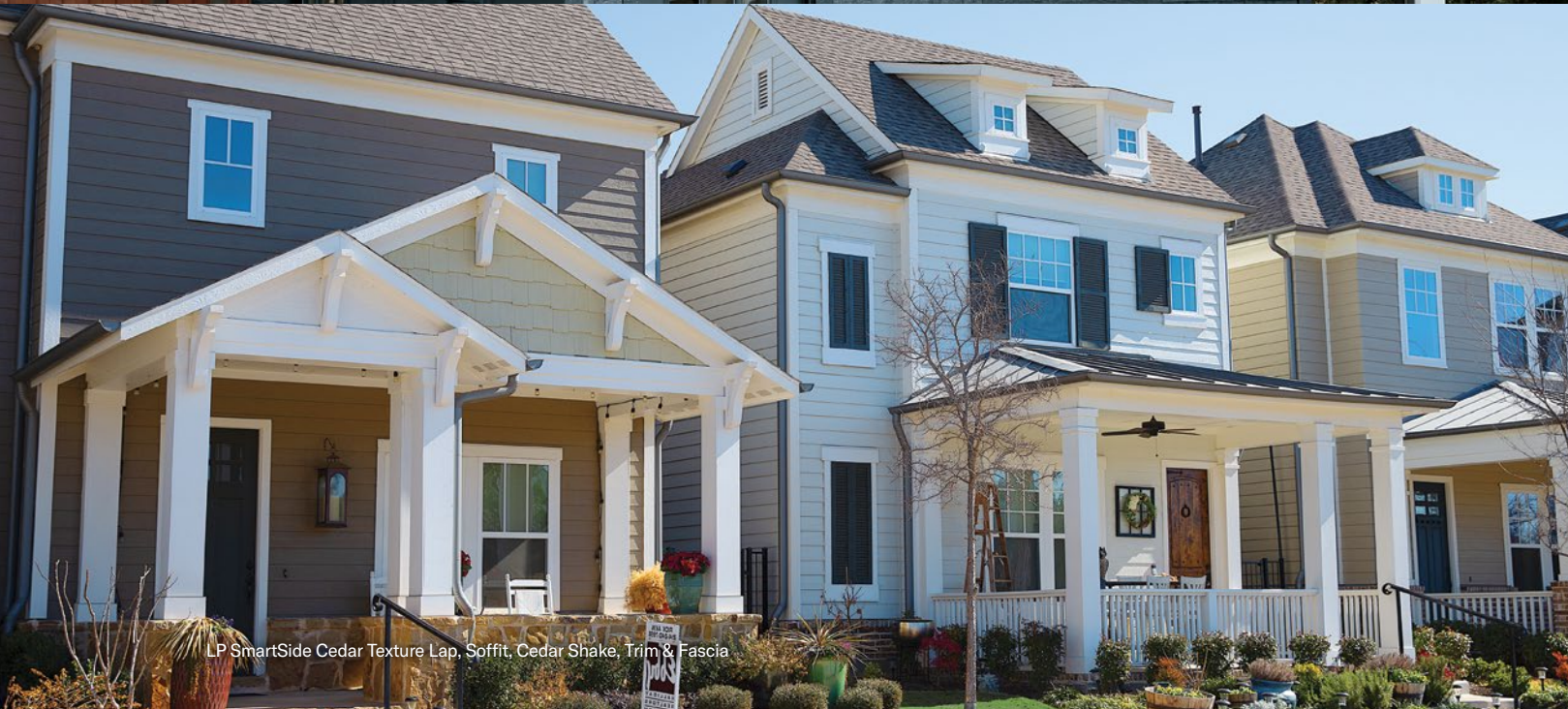
Featured: LP SmartSide ExpertFinish Cedar Texture Shakes, Trim, Fascia, Soffit & Accessories in Abyss Black
